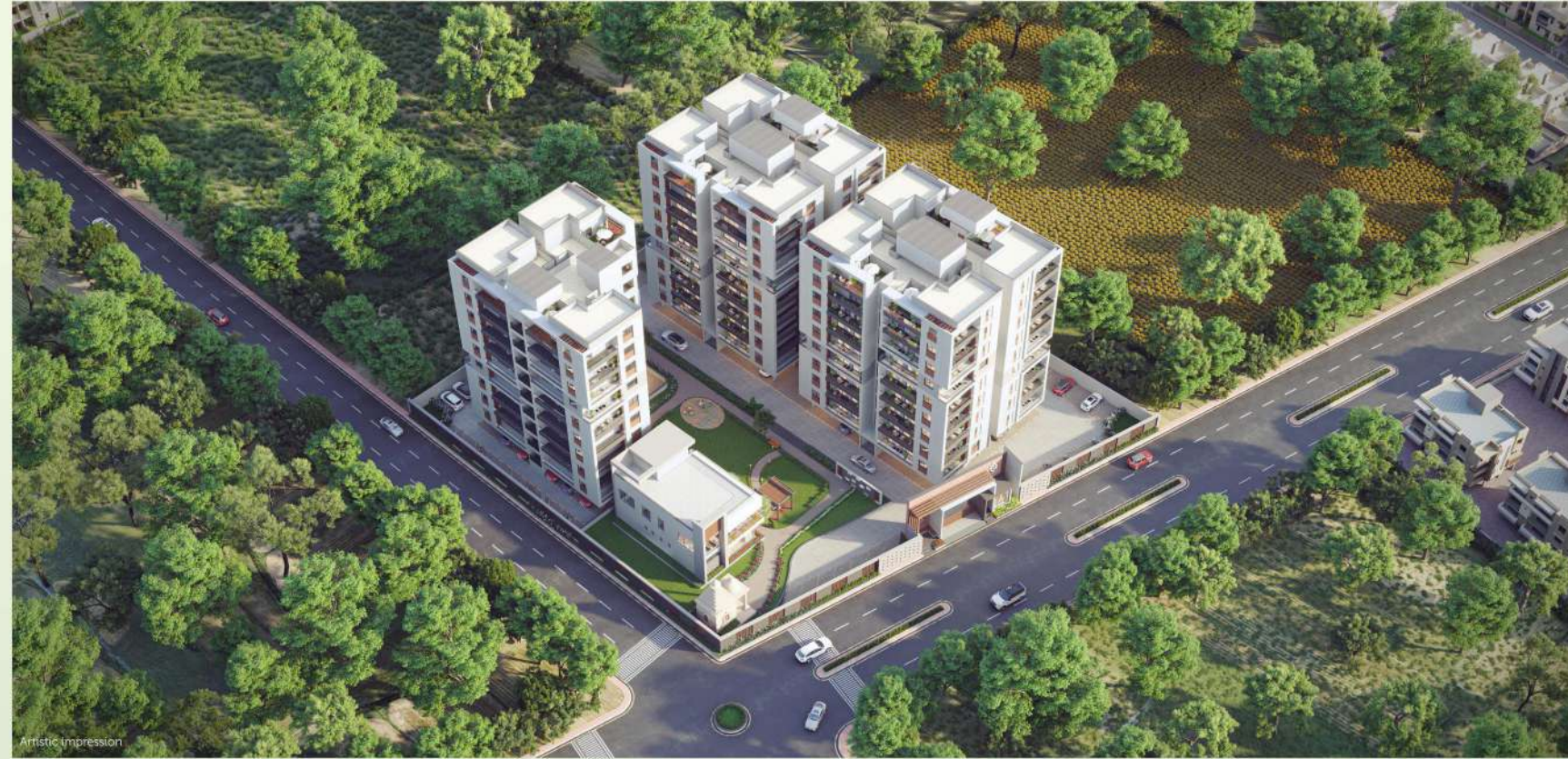
Site Address : Green City Extension Near SPS Rohit nagar, Bawadiya Kalan, Bhopal 462026
